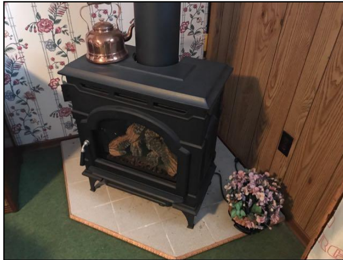
14. System was shut off
