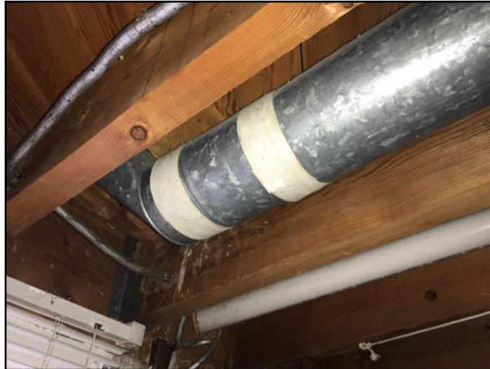
16. The duct work in the basement was found to...
